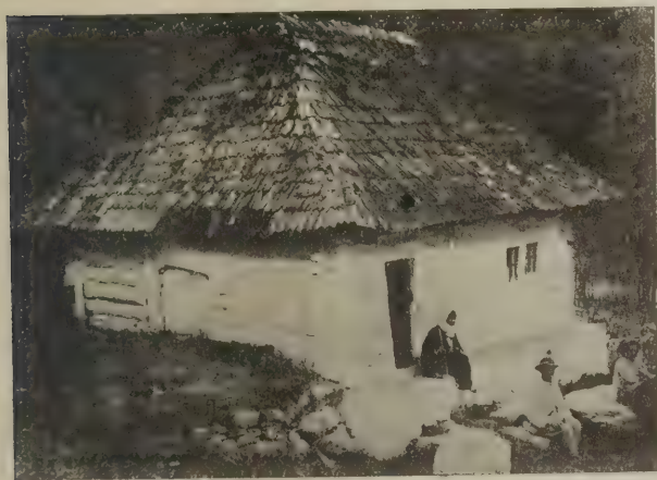
A PEASANT HOME IN THE CARPATHIAN MOUNTAINS. THIS HUT IS OF CHINKED LOGS, WHITEWASHED AND THATCHED. TO THE CARPATHIAN MOUNTAINEERS A "PLACE IN THE SUN" MEANS JUST A DOORSTEP ON WHICH TO SIT AFTER THE DAY'S WORK IS DONE. THE WAR BROUGHT NOTHING BUT FAMINE AND DISTRESS TO THESE SIMPLE FOLK, AND IT WAS AMONG THEM THAT THE AMERICAN RED CROSS RELIEF EFFORT IN THE BALKANS WAS CONCENTRATED
